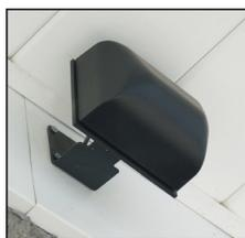
**Motion Detector-** Turns the air curtain on when sensors detect motion so that the air curtain is already operating before door is opened.
