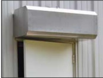
**WALL MOUNT** -- Back side of air curtain has 4 mounting holes capable of accepting four 3/8 mounting bolts or lags, with washers (use these holes only for mounting). Mark and pre-drill mounting surface accurately. A long extension and ratchet will negate the need to remove the motor-blower plate when installing.
