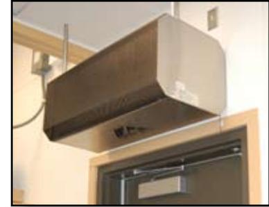
**THREADED ROD (by others)** -- Unit has four 3/8-16 threaded inserts for installing one end of threaded rods. The other ends of the threaded rods can be attached to the ceiling. Threaded rod should not extend more than 3/4 inch into air curtain.
