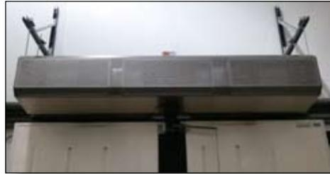
**BRACKETS** -- Mounting brackets (also called knee, angle or L-brackets) can be flush to the wall or constructed to account for a projection from the wall. For proper size brackets measure standoff distance from wall to back of where air curtain will be.
