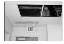
Attach the intake/discharge grille to the bottom of the air curtain. The grille is larger than the air curtain to cover the gaps between the air curtain and ceiling.
