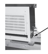
The air curtain is lagged to the bottom of the crate frame. Remove screws. Unit is now ready for installation.
