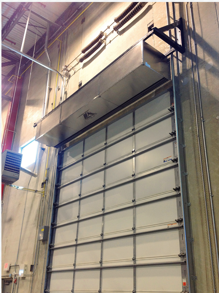
Model BPA | Brackets; High Turn-Back track Door.
