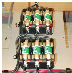
Single Point Power Connection
