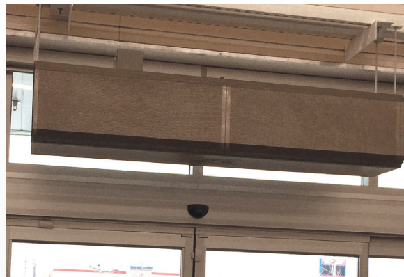
Model CED | Top Mount (Threaded Rods)
