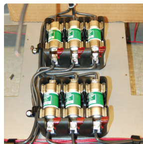
Single Point Power Connection
