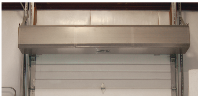
Model ETD | Top Mount, Brackets
