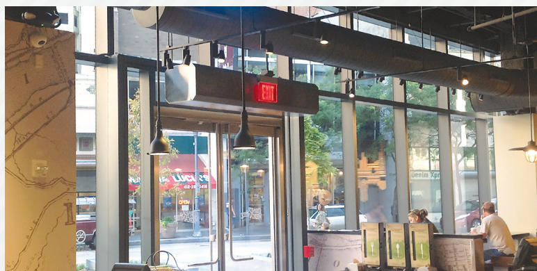
ECE-E | Top Mount (Threaded Rod)
